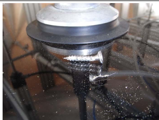
Picture 3 One of the screws used to fix the collector.
